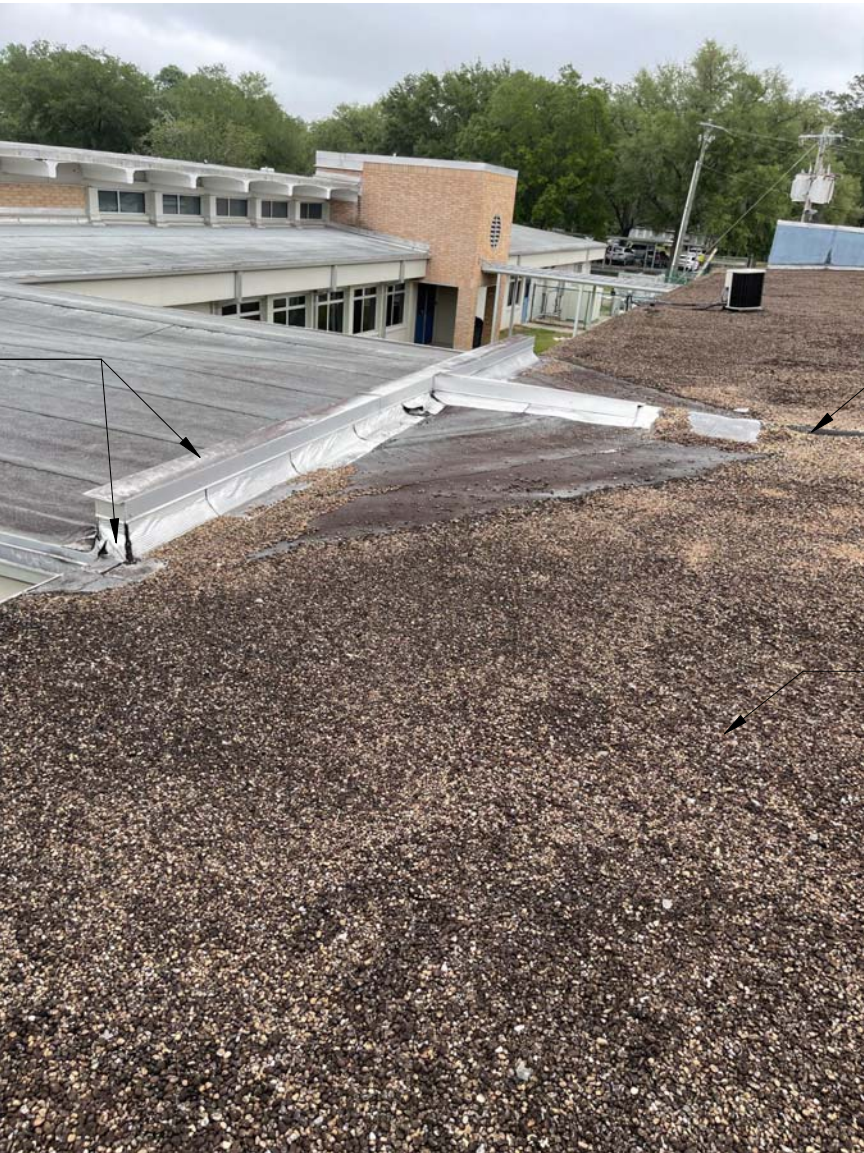
Existing Roof Curb/Cricket Transition
