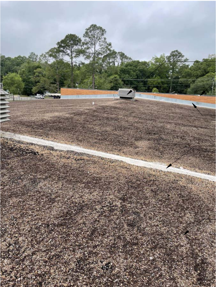
Existing Expansion Joint - West End
