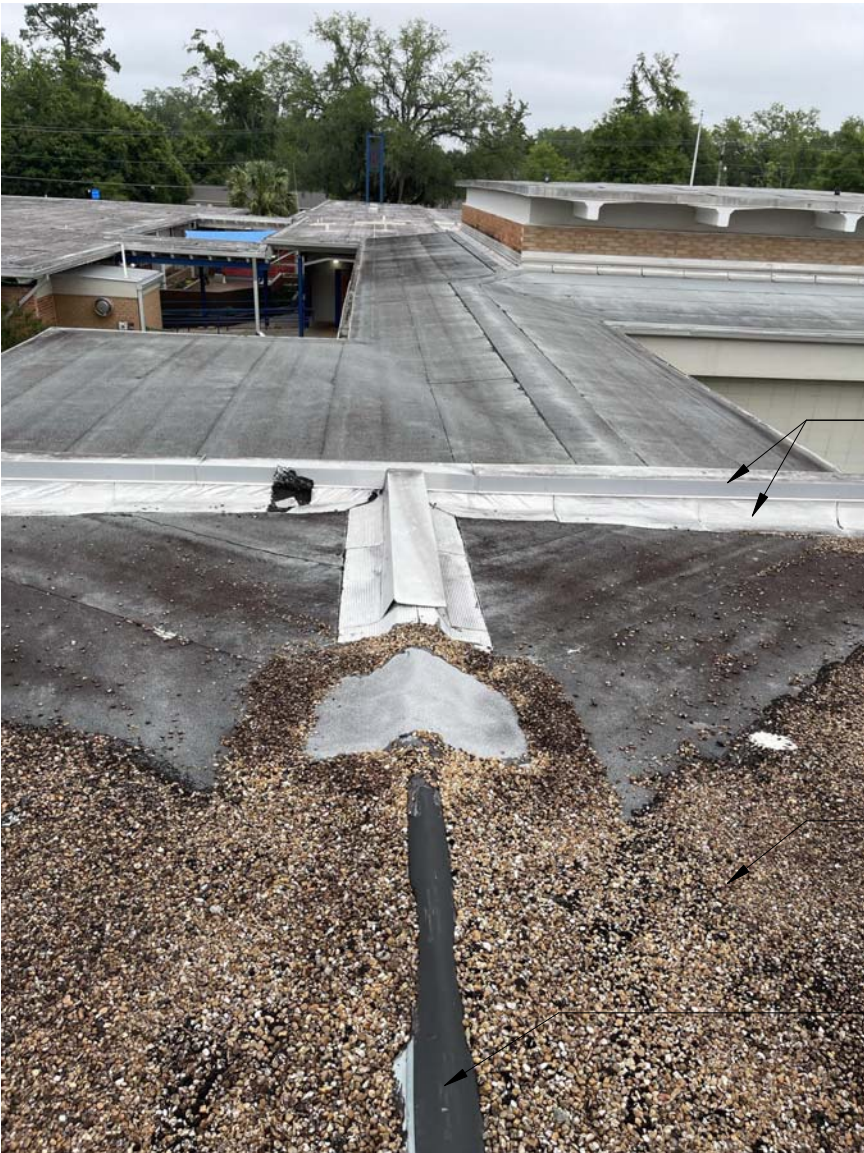
Existing Expansion Joint - East End
