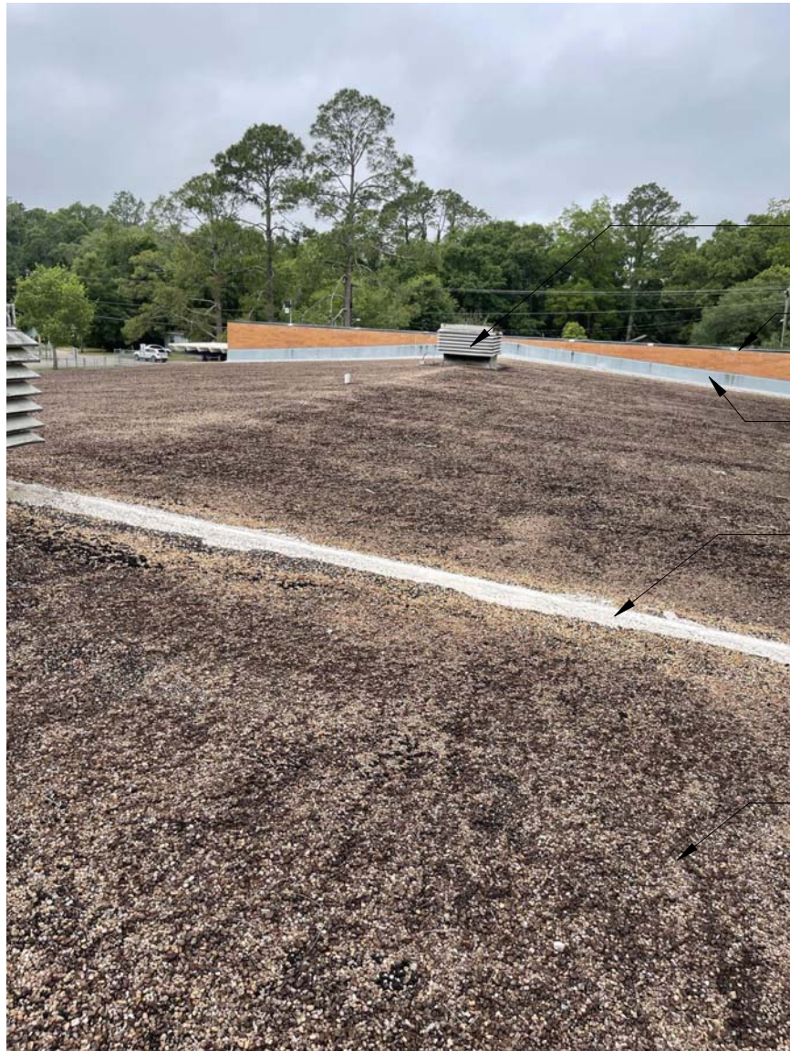
Existing Expansion Joint - West End
