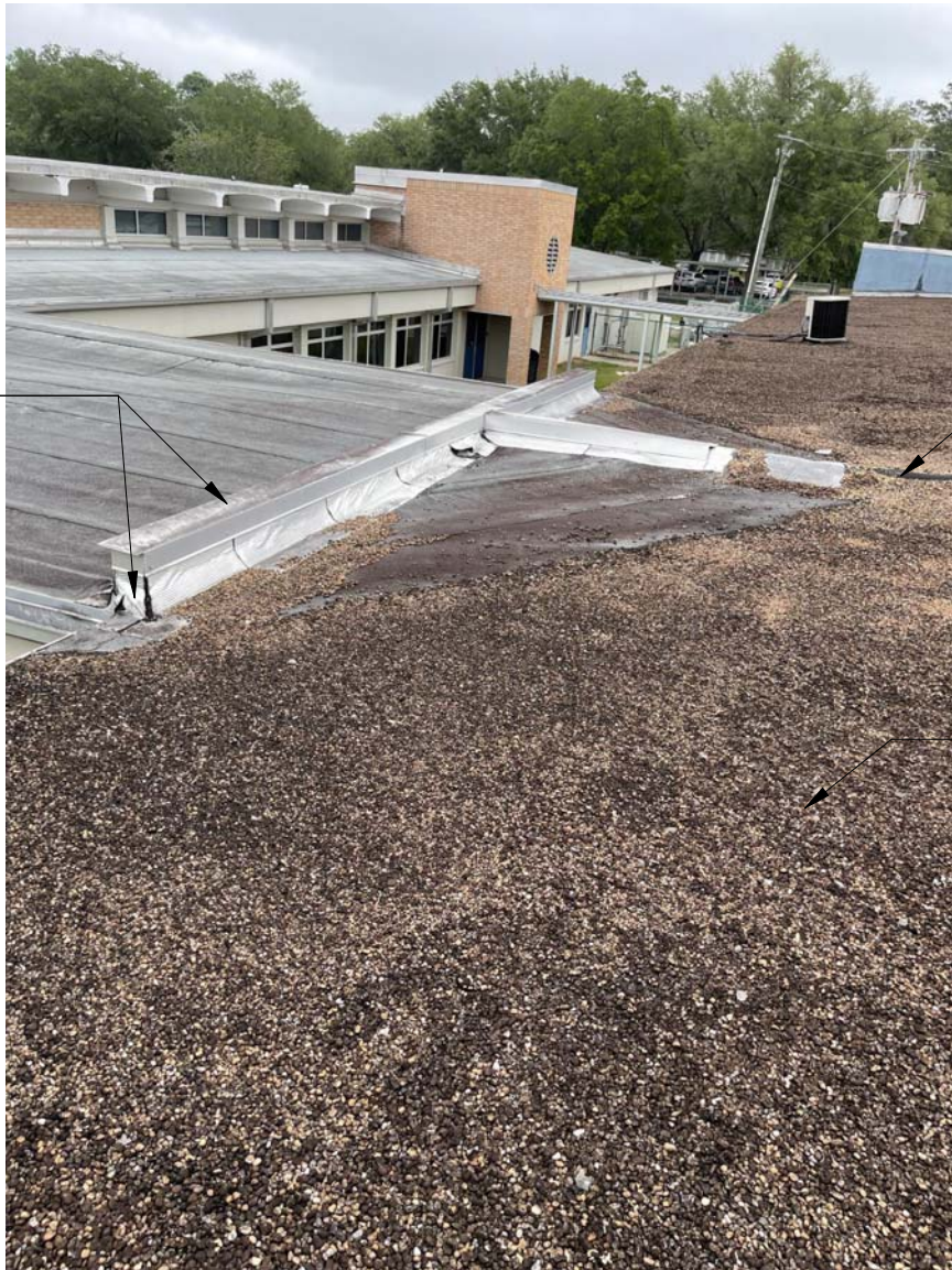
Existing Roof Curb/Cricket Transition
